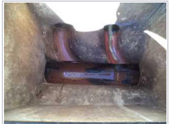
Drains clear where visible
