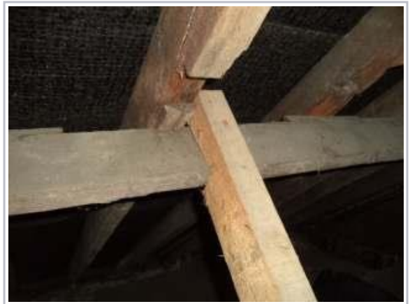
Inadequate purlin
