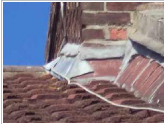
Basic tiled chimney flashings
