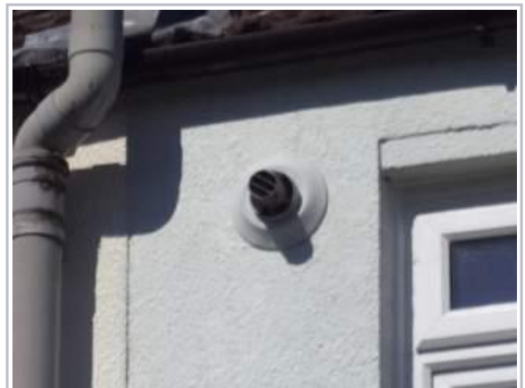
Boiler flue
