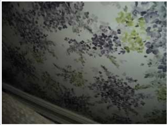
Unvented chimney breast
