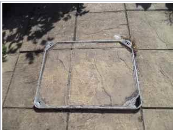
Inspection chamber cover
