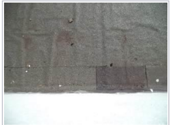
Flat roof has been patch repaired
