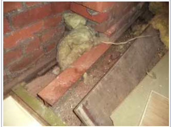
Chimney in loft supported on RSJ
