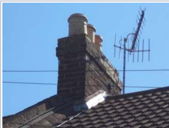
Front of chimney
