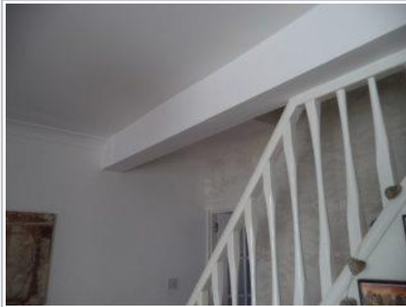
Wall removed in dining room
