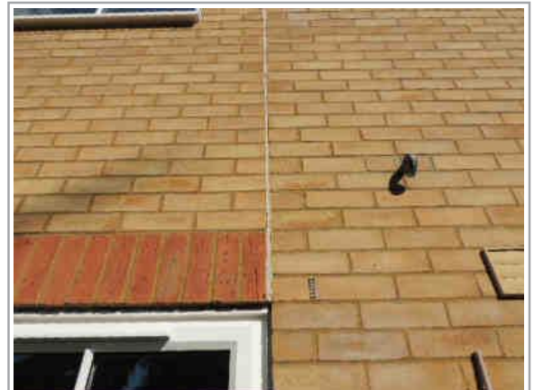
Correct expansion joint
