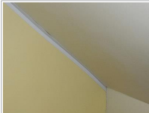
Shrinkage cracks
