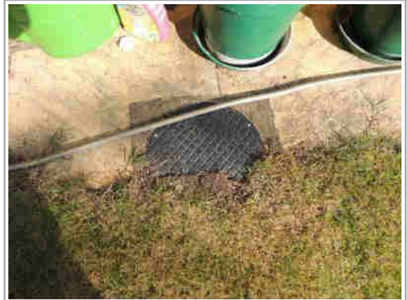
Cover grown over and screwed shut
