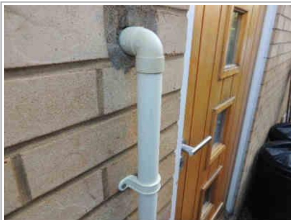
Uninsulated condenser pipe
