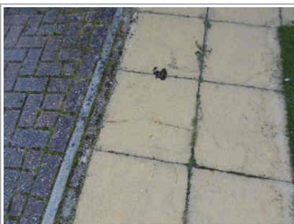
Cracked slabs
