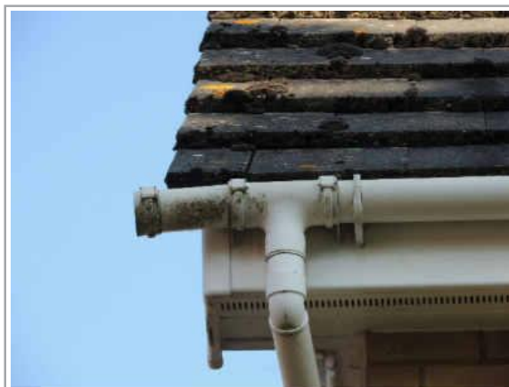
Re-align gutter
