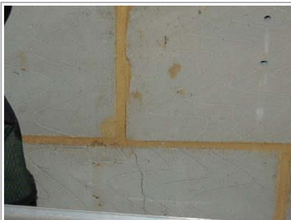
Cracks in garage
