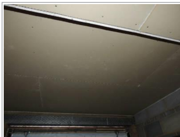
No hatch to roof void
